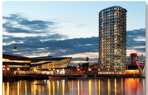
Pump Tower Royal Victoria Dock, London
